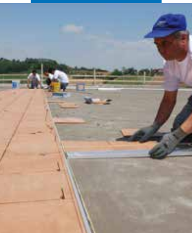
Installing ceramic with Kerabond + Isolastic
