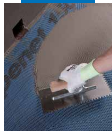
Laying Mapelastic on Mapetex 150
