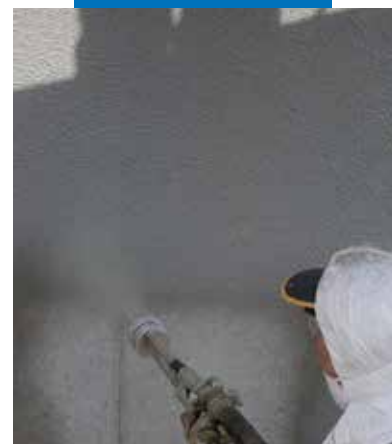
Example of Mapelastic applied on a viaduct by spraying
