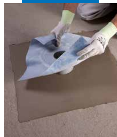
Application of Drain Vertical on Mapelastic
