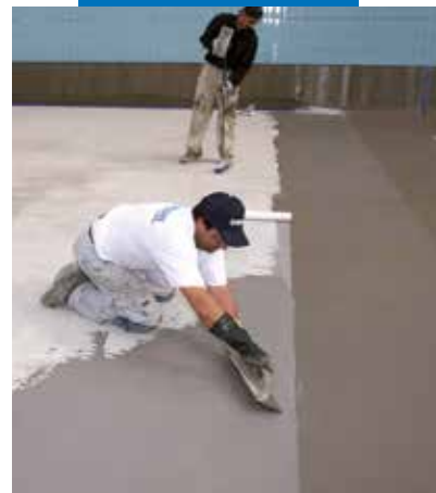
Waterproofing a swimming pool with Mapelastic
