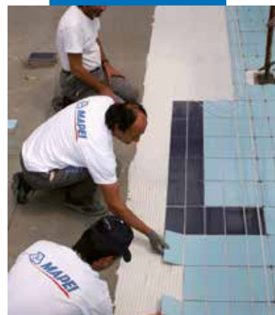
Laying ceramic tiles on Mapelastic in a swimming pool
