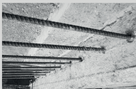
Post-Installed Rebar Connection
