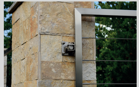
Gates, Railings, Fencing
